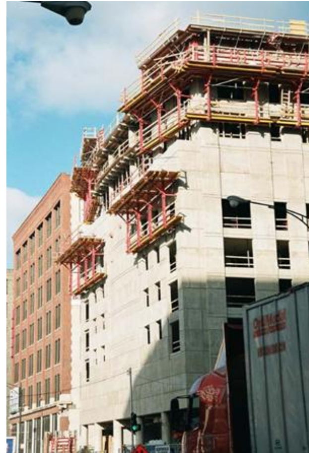
Grand Orleans, Chicago, IL Contractor: Goebel Forming
