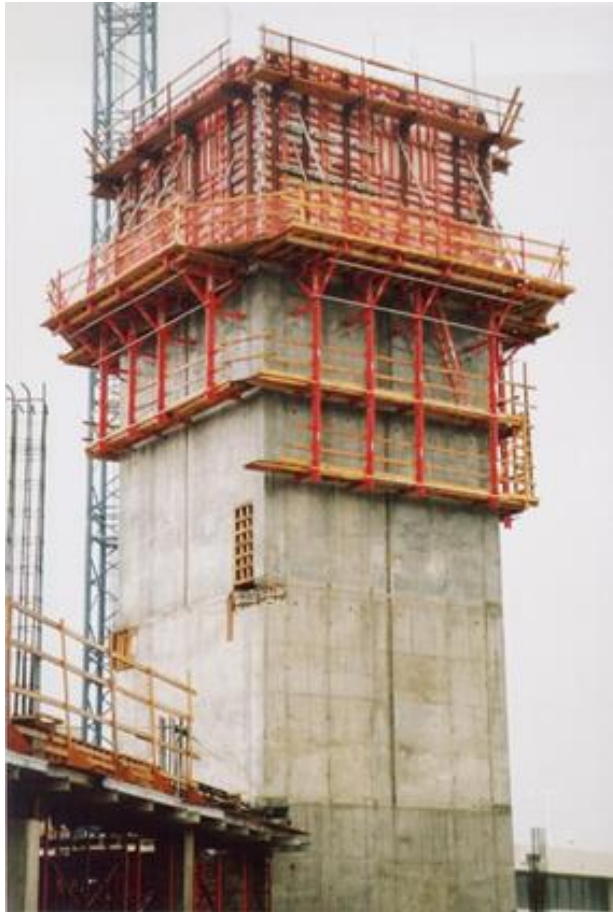
Airport Control Tower, Miami, FL Contractor: Baker Concrete
